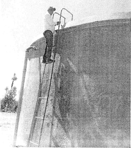
The water tank at the Busakala Water Treatment Plant
