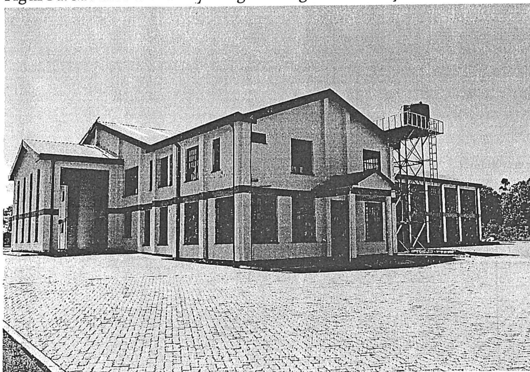
Figure 2: Milk Processing Plant in Webuye
