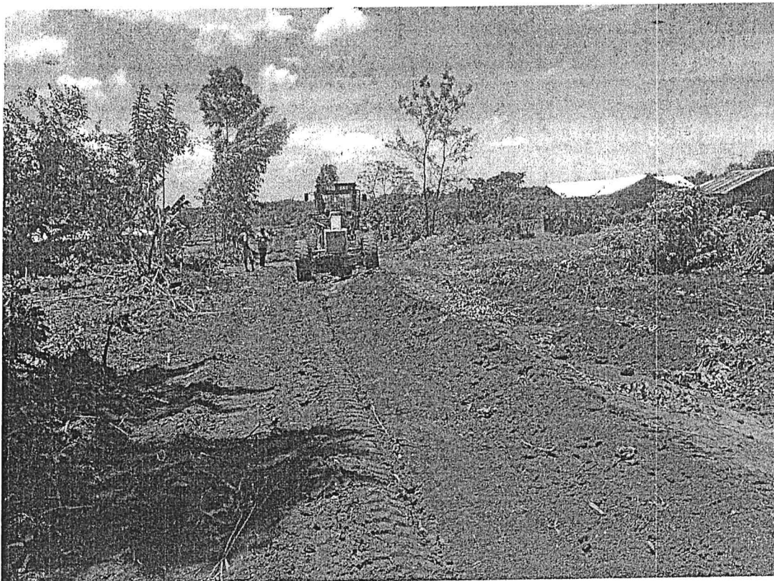
Grading of the Dumpsite Access Road
