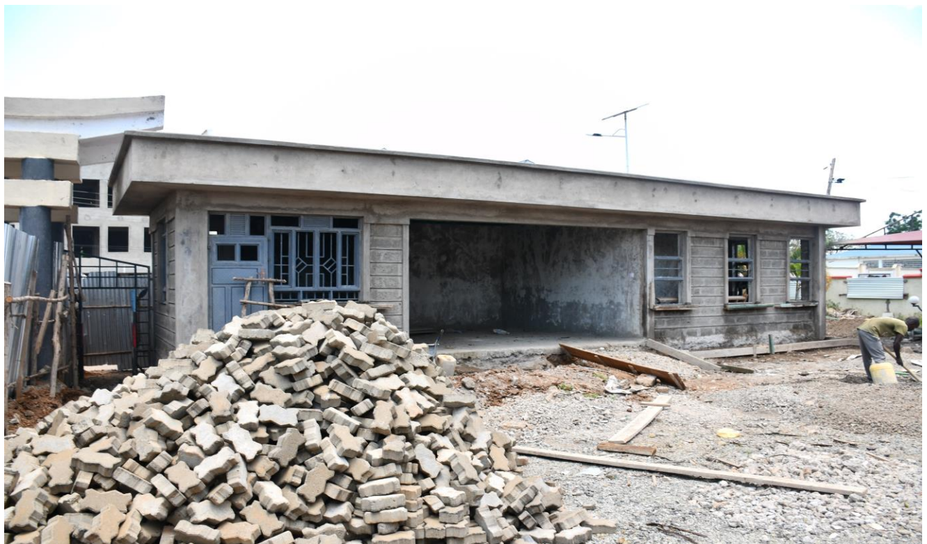
Picture 12: Construction of Visitor's Waiting Bay
