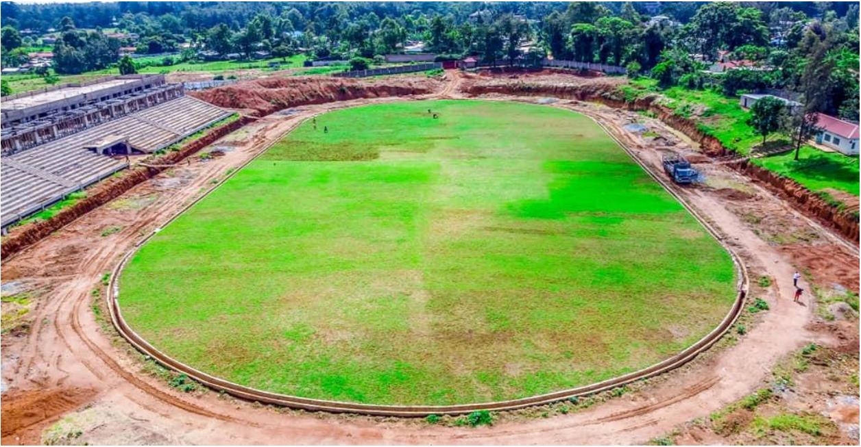
Upgrading of Masinde Muliro stadium in Kanduyi
