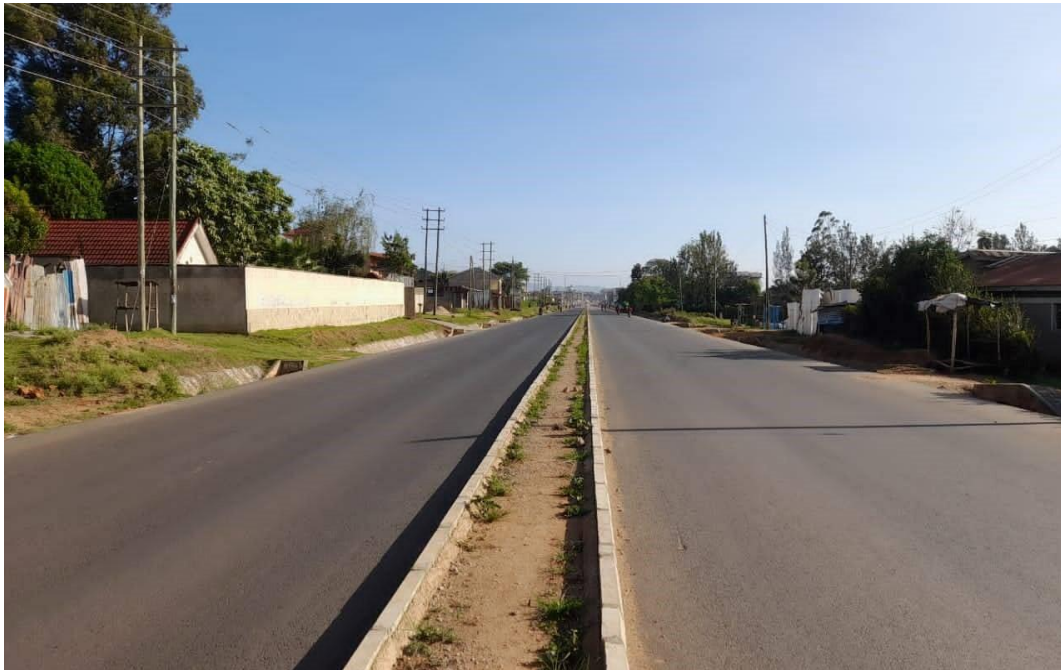
Figure 4: 6.5km Sangalo Junction – Kanduyi Dual carriageway
