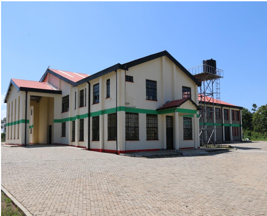
Figure 2: Milk Processing Plant in Webuye
