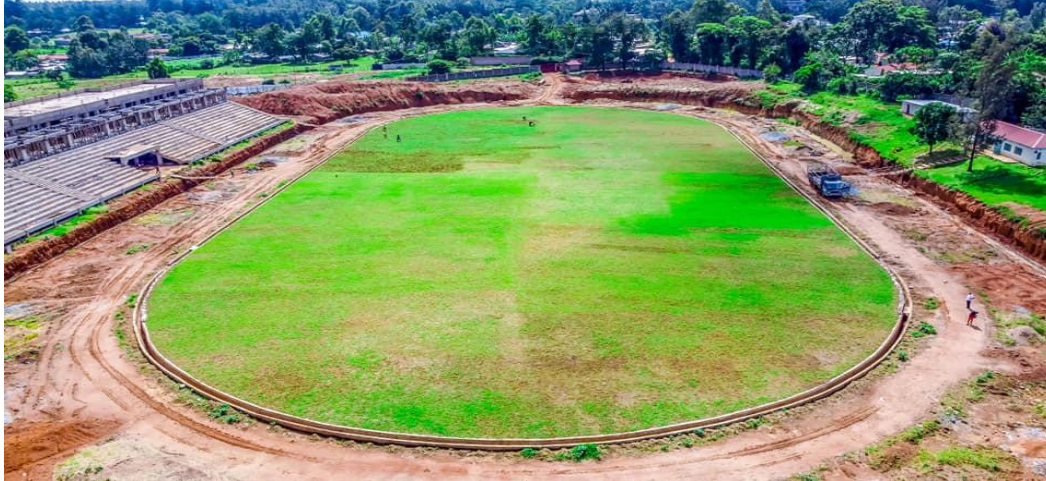
Figure 3: Upgrading of Masinde Muliro Stadium in Kanduyi
